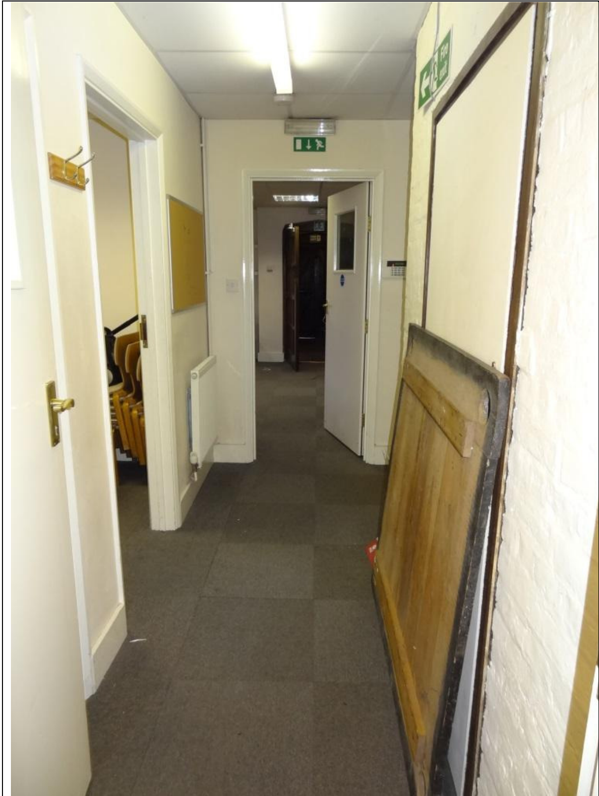
Fig. 12 Hall ancillary room
