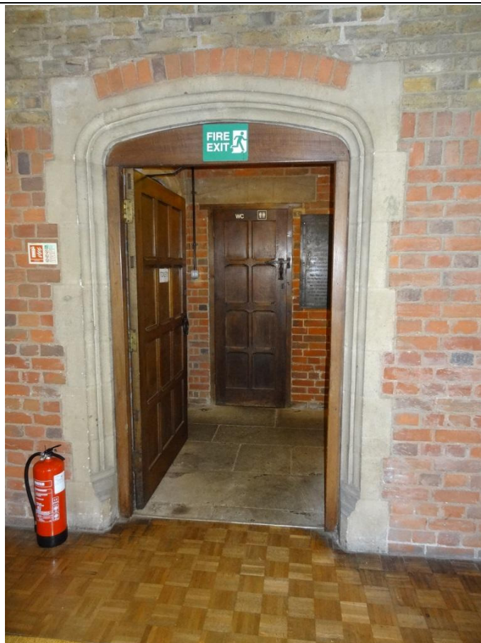
Fig. 4 Door connecting church to side entrance lobby (D.02 & D.03 in background)
