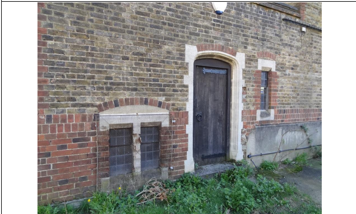
Fig. 14 Existing entrance to Former Boiler Room
