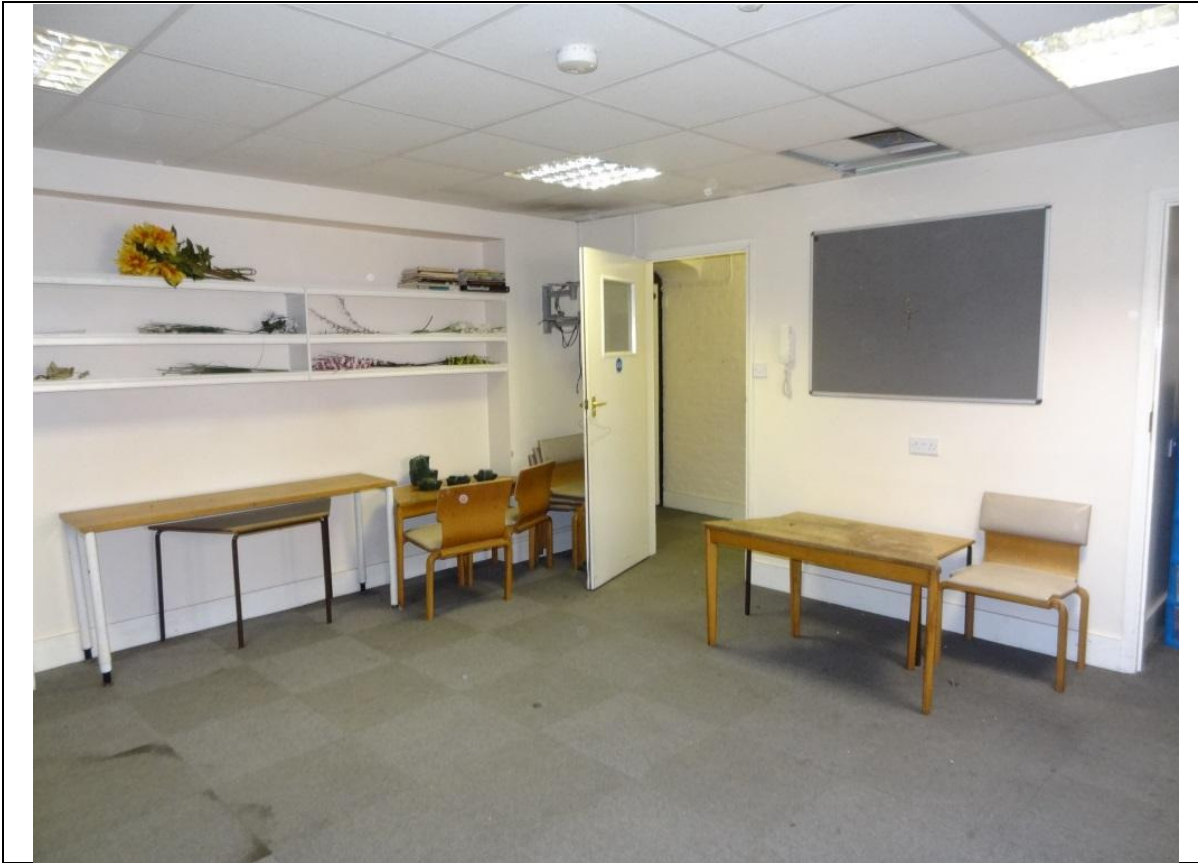
Fig. 8 Hall looking east towards D.07 & D.08
