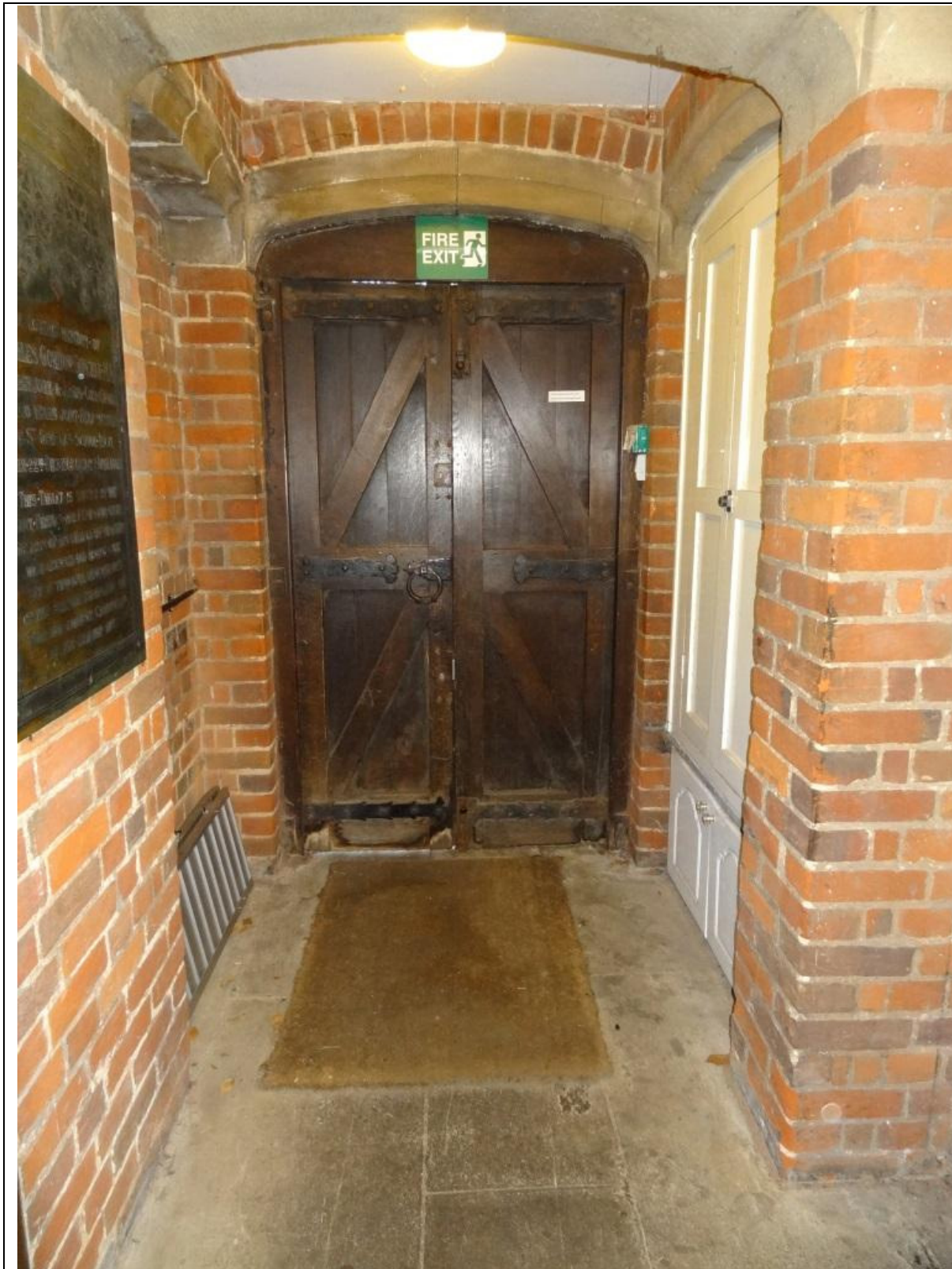
Fig. 1 Side entrance Lobby – External doors (D.01)
