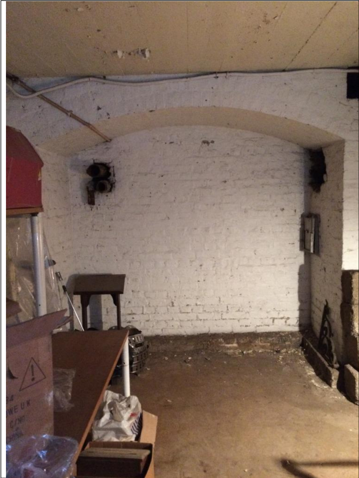
Fig. 15 Former Boiler Room
