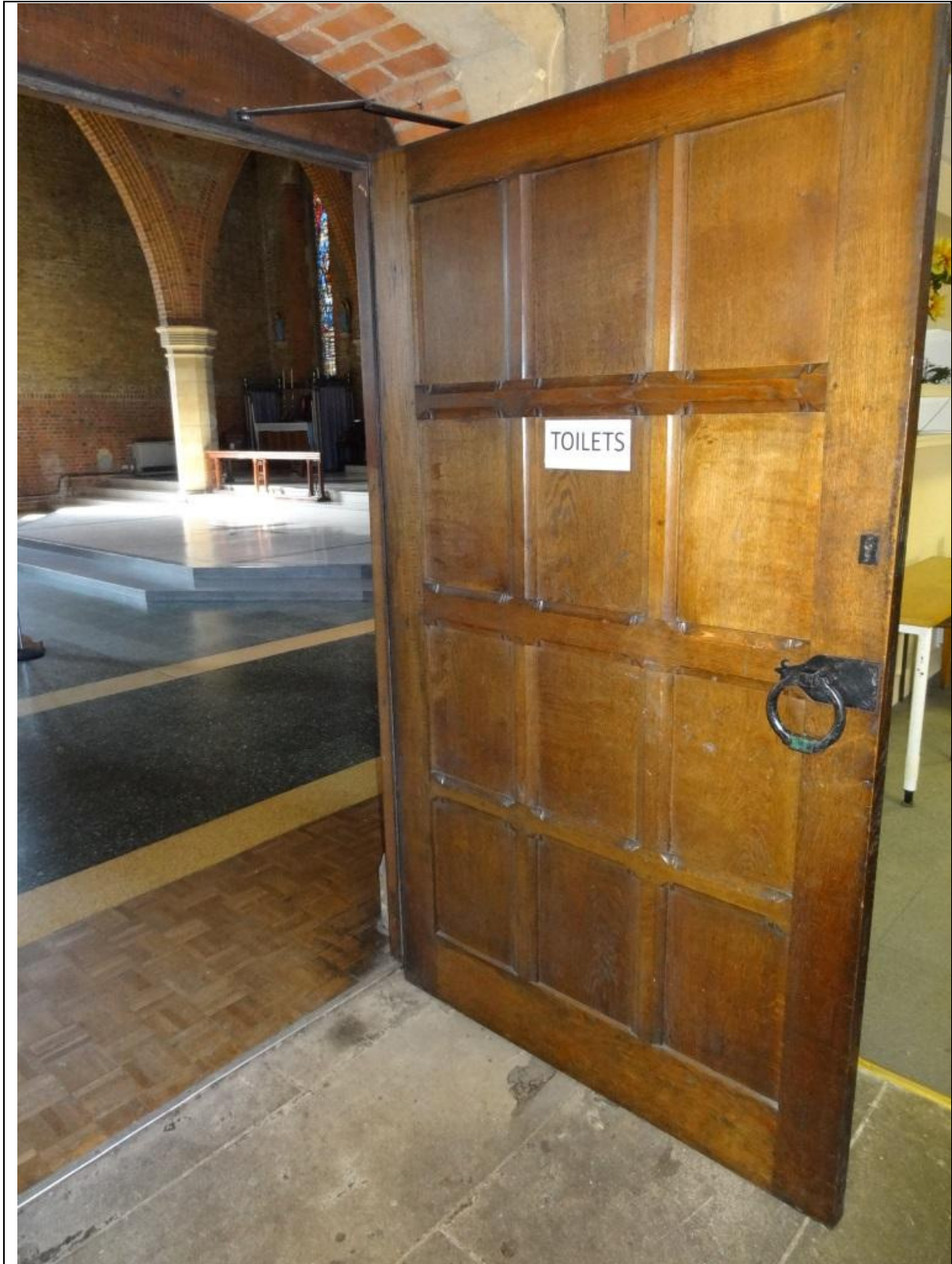
Fig. 2 – Door connecting side entrance lobby to church (D.02)
