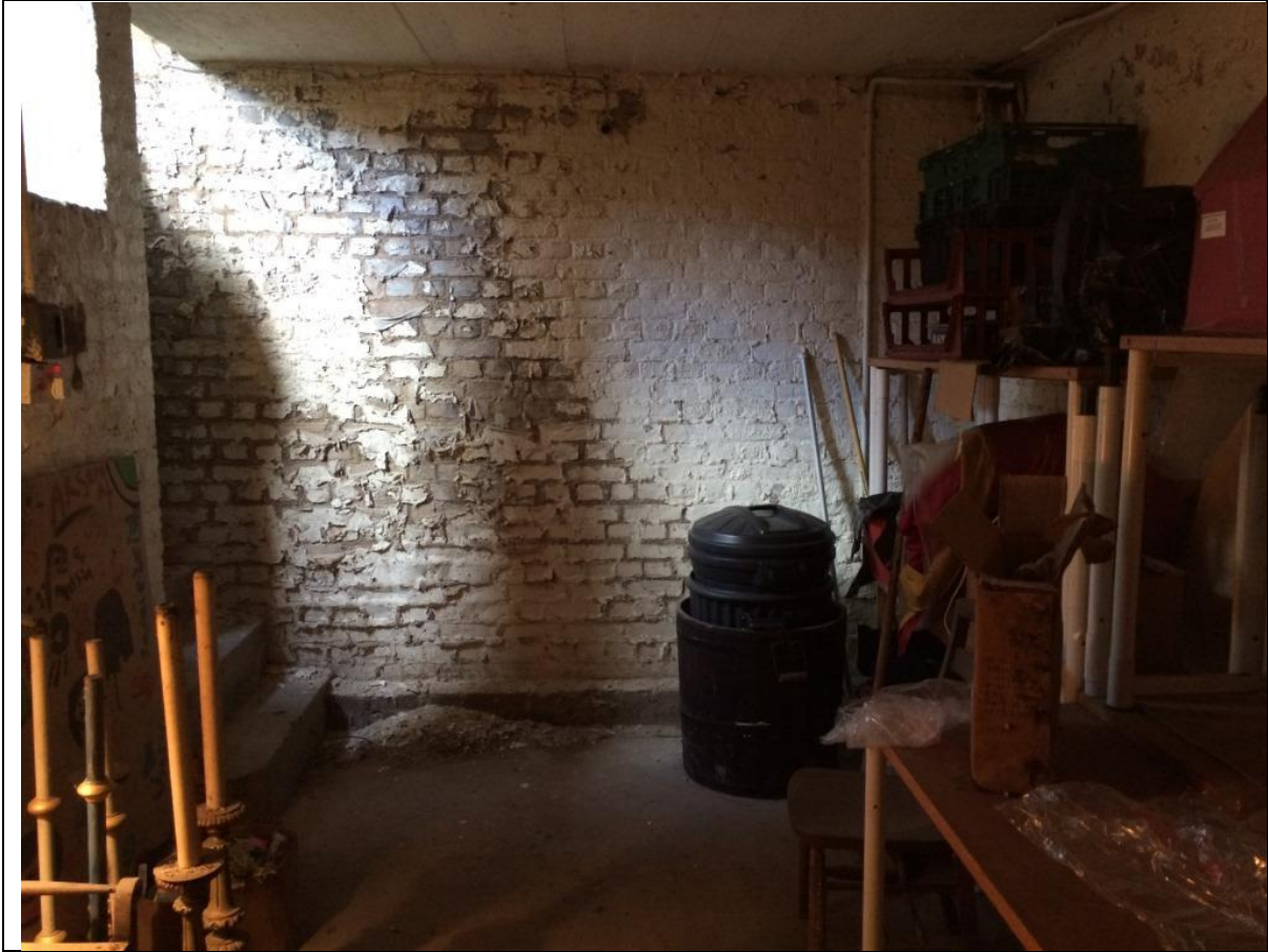
Fig.16 Former Boiler Room
