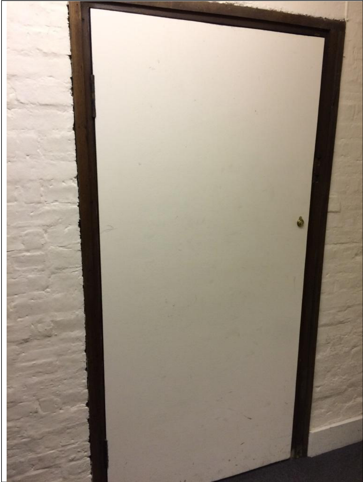
Fig.17 Fire-proof boarding to existing door
