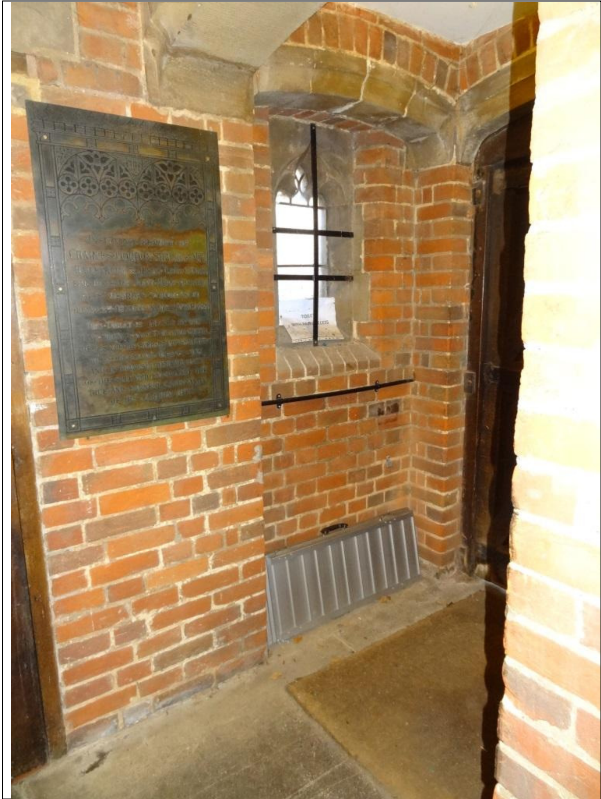
Fig. 5 Side entrance lobby
