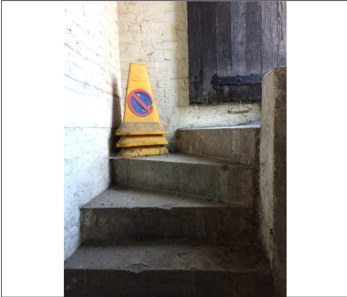
Fig. 13 Top of steps up from Former Boiler Room
